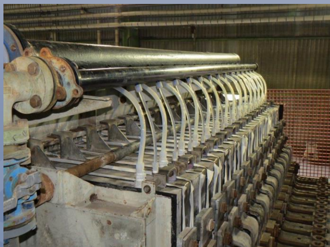
6" Double-Boss P-72 Header with FRP Overlay
